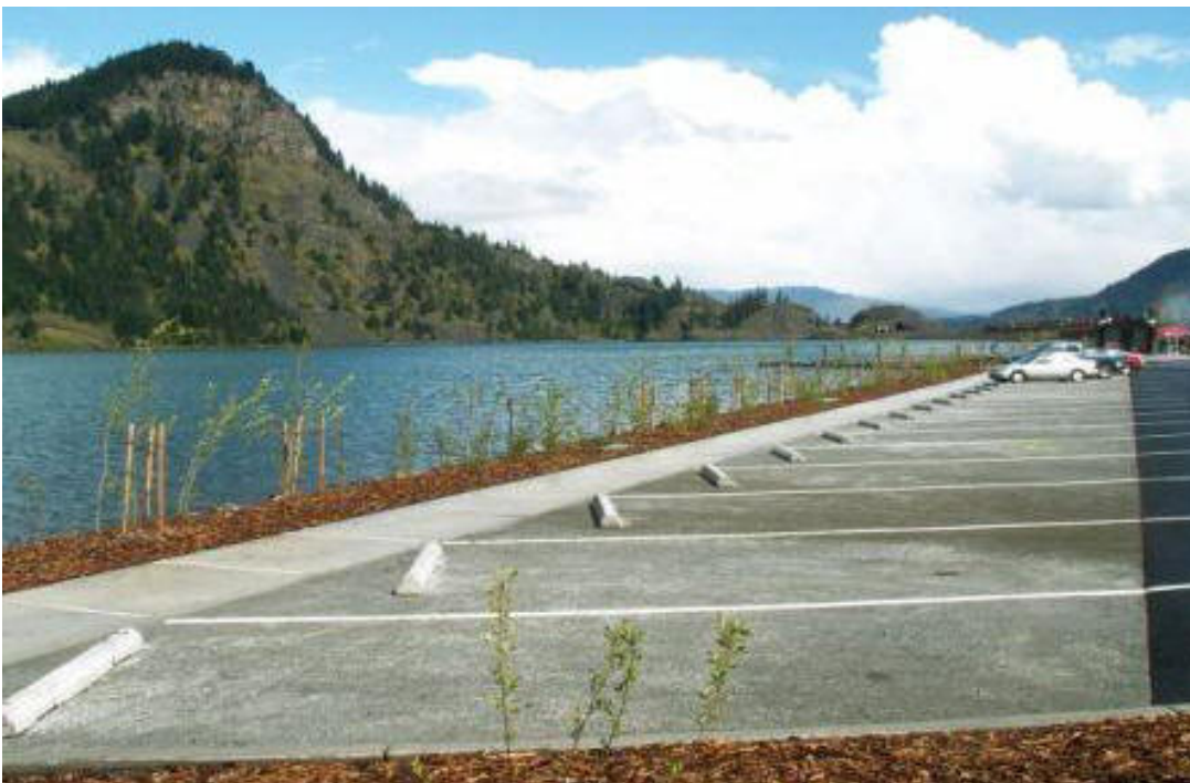
Figure 3 -Pervious pavement is a unique and effective means of addressing environmental issues. Image source: http://www.perviouspavement.org/
